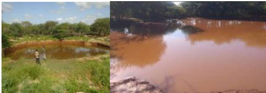
Figure 4. New pond in Adela Kebele Goje sub-site (left) and Ardakelo kolosite (right) in Raytu
