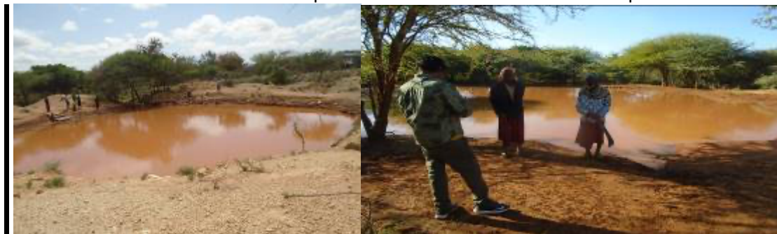
Figure 5: Structure with cattle trough constructed in Adela kebele (left) and Arda Kalo kebele maintainace pond, Rayitu
