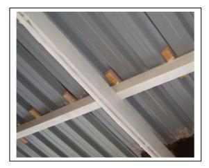
Phase I showed that poor nailing of roof sheets sometimes caused localised leaking at nail points.
