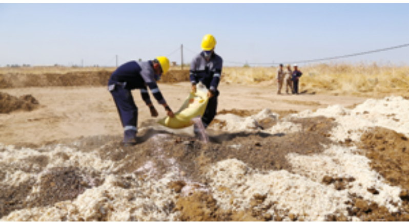
Preparing a biological treatment cell for oil contaminated soil in Kirkuk, Iraq. Photo: UN Environment
