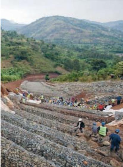
From the construction of the power plant in Bogoye, which was opened by Erik Solheim, Minister of International Development, in autumn 2009. Steps are built in the overflow weir by placing rocks in 'chicken wire'. The weir is important for leading water away when the flow of water in the channel is particularly strong. (Photo: Ken Opprann)
