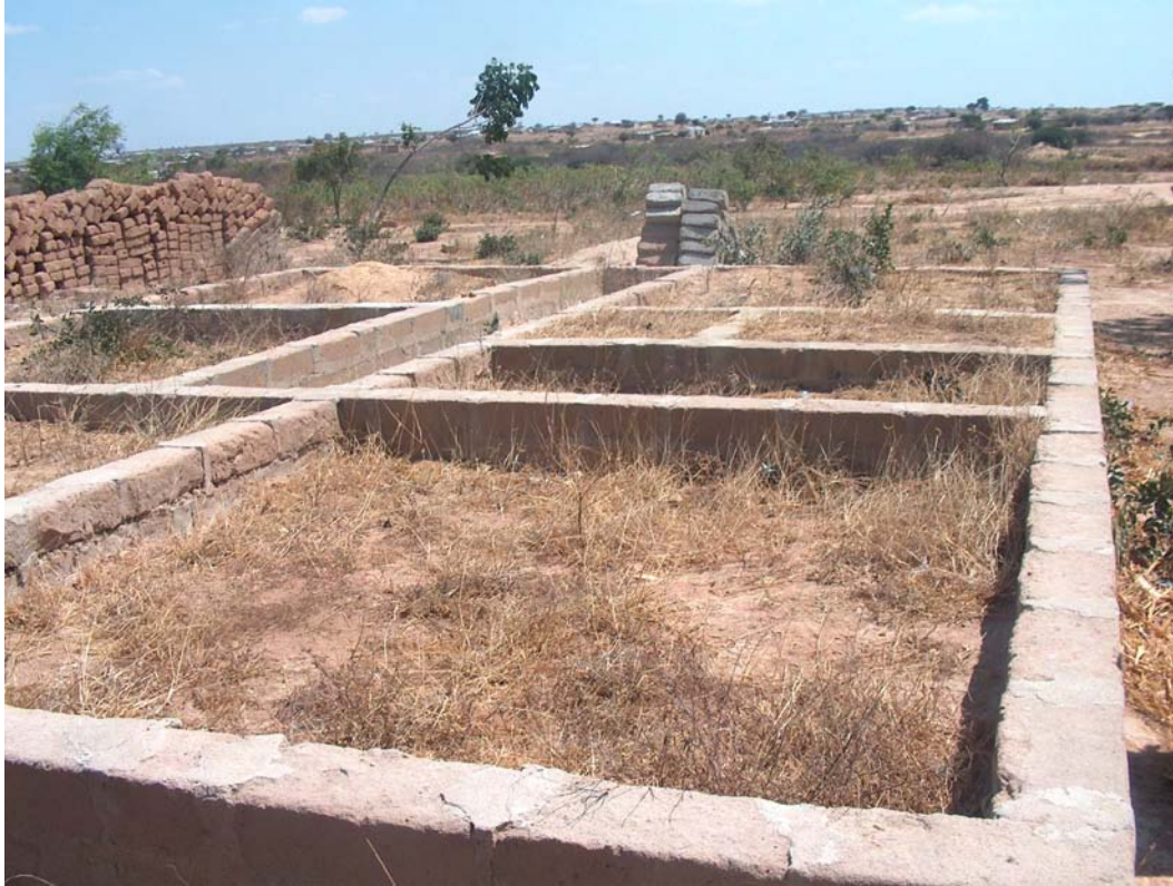
Fig. 2.3 Construction at foundation level
