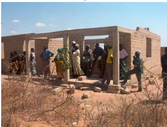
Fig. 2.4 Construction using stabilised soil blocks
