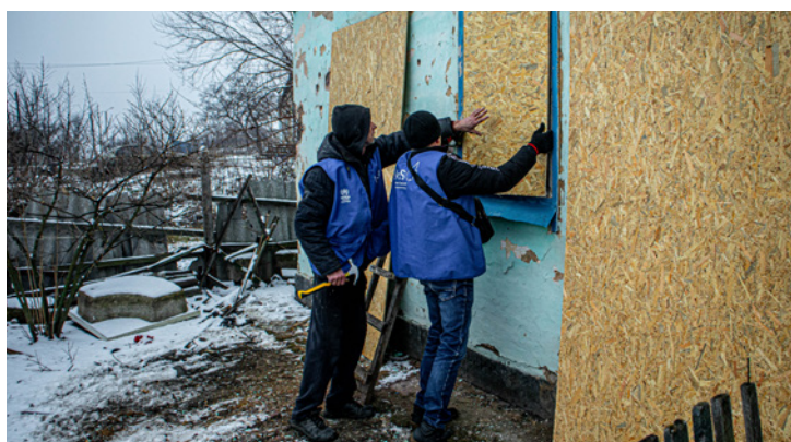
↑ UNHCR's partner organisation Angels of Salvation helps residents near the front line in the Donetsk region repair their war-damaged homes. | Photo: Oleksii Hutnyk, Angels of Salvation
