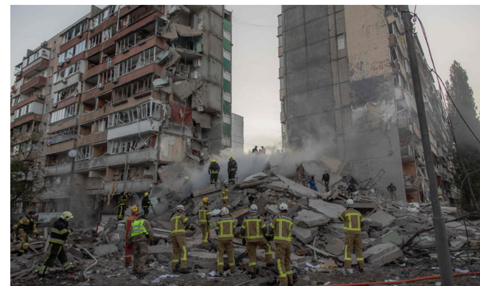
↑ Rescuers work at a residential building partially destroyed following Russian drone and missile strikes in Kyiv in the morning of May 14, 2026. | Photo: Roman Pilipey, AFP/NTB
